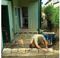
**Sandstone steppers:** sawn sandstone slabs provide stable stepping stones with a touch of class. Random sizes staggered through the lawn appear to dissipate then regroup in the form of a stacked water feature.
