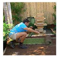
**Lawn:** a fine-leaved winter green couch lawn was laid over turf underlay to provide a soft spot to enjoy the sun. A 90/10 underlay mix (90% coarse washed sand/10% black soil) was spread to a depth of 50mm to improve drainage and provide some additional nutrients to help establish the new turf. **Blitz Tipz:** If you have a sloping lawn, lay rolls of turf across the slope to avoid water running between the rolls and washing out your soil.
