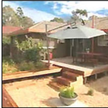
The cantilevered boardwalk was constructed from 90x90mm treated pine posts, 140x140mm treated pine bearers and 90x45 joists. Merbau hardwood decking was laid.
