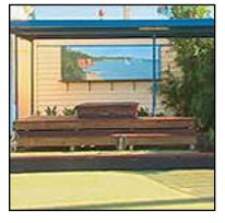
**Barbecue:** Jamie built a support for the new barbecue with lightweight, aerated concrete blocks. Block walls built 800mm high support both the barbecue and pavers to act as a servery on either side. A bagged finish of yellow brickies sand and off-white cement provides an attractive top coat to the barbecue. Grey coloured caulk disguises the joins between pavers on either side of the barbecue and prevents food or grease from settling between pavers.
