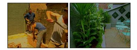
**Step 1** Check existing walls and floor are level. If the surroundings are not level you will have to adjust your new work accordingly. Use a string line to mark out the position of the garden bed walls.
