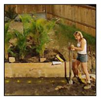
**Retaining wall:** Nigel and Jamie built a low retaining wall using treated pine sleepers (2400x200x75mm). Posts were installed vertically in-ground to 600mm deep. They were surrounded with concrete support sleepers stacked horizontally and connected with galvanised cup head bolts (200mm long).
