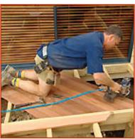
Laying decking boards at a 45-degree angle will increase the amount of waste (as opposed to laying them perpendicular to the joists) and will need to be taken into account when ordering your timber.
