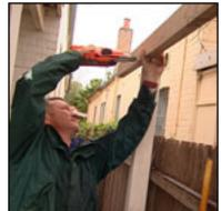
Climber framework: 11 posts (H4 90 x 90mm) were installed by Scott vertically in-ground in rapid setting concrete immediately in front of the fence. A top rail (90x45mm) connected to the top face of the posts acts as a brace to prevent the posts from sagging when under tension. A row of wires was attached between the posts with saddles and tensioned with galvanized gripples and a gripple tool. *Blitz Tipz*: In small spaces, use vertical structures to provide another growing area.
