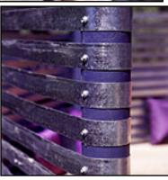
**Blitz Tipz** To create a curved treated timber edge saw a third of the way through the timber at regular intervals and bend around hardwood pegs before nailing into place.
