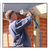
**Arbour:** Scott built an open-topped arbour to create a link between the house and garden (see pics above). Treated pine posts (H4, 90x90mm) were installed in-ground in rapid set concrete. The posts support a beam (140x45mm) bolted in place with galvanised cup head bolts. The entire structure was painted with an exterior low sheen acrylic paint. **Blitz Tipz:** Pre-cut decorative ends before clamping beams in place to enable safe drilling of holes for bolts.
