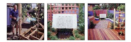
**Water feature:** a food grade polyethylene stock trough was laid in a sand lined hole dug to shape in the garden. All voids were backfilled with coarse washed river sand. A sheet of carved granite was suspended across the trough and supported by sandstone blocks on either side. A cascade of water runs over the granite feature into the pond below and is recirculated by a low voltage submersible pump.
