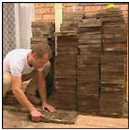
**Paving:** Nigel lifted the tired old paving and laid large format sandstone pavers with a small unit paver surround to provide a level entertaining area. Large format sandstone pavers (400x400x35mm) from Sareensone add a touch of class and lightness to the courtyard and beneath the pergola.
