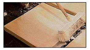
Step 1 Spread a 50mm layer of crusher dust (or river sand) over the area and level.
