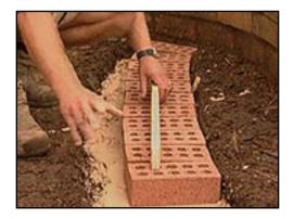
Laying bricks along a contour means that they are at an angle to each other requiring more mortar at one end than the
