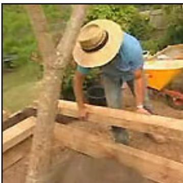
**Planter boxes:** Jamie used sleepers to create planter boxes for the frangipani, making sure of a sound level base to lay sleepers on edge. Our box height was 470mm and this was two sleepers on edge and a capping sleeper laid flat for seating, with the ends cut at 45 degrees to give a mitred finish.
