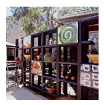
**Shelving:** treated pine posts (H4, 90x90mm) installed inground in concrete combined with treated pine rails (70x45mm) and hardwood shelving (290x19mm) make an artistic feature wall and outdoor shelving unit. Builder Scott Cam has combined these elements to create a privacy wall that doubles as a display unit for the sheet metal art works and display pots. Steel bar stools and an adjustable red gum bar provide the perfect place to relax on a summer's evening.
