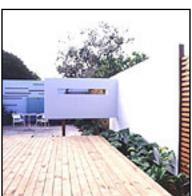
**Feature walls:** feature walls were erected to divide the garden into two rooms and to add interest. Timber posts (100x100mm) installed in the ground in concrete carry a pine frame (70x35mm). Harditex base sheets (2400x1200mm, 2400x900mm, 9mm thickness) were attached with stud adhesive and clouts.
