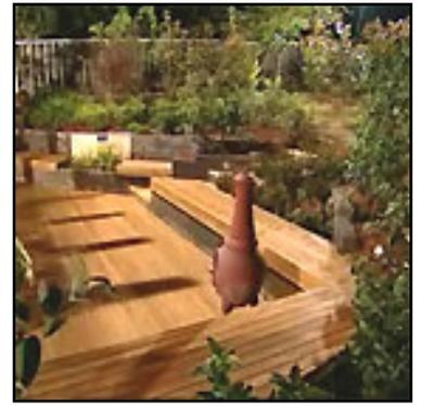
**The water feature:** Using three pieces of channel drain Jamie and the team created a cascading water feature by laying the channel on three different levels. Acqua bisazza tiles were then glued and grouted in the channel. The water trickled down a wall and into the existing reservoir which had three coats of water proofing membrane. The wall face was clad with vanilla split stone marble. We applied three coats of a waterproofing membrane to the reservoir.
