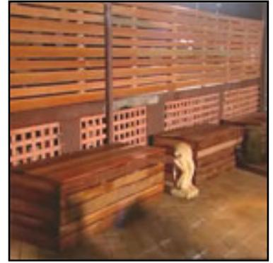
**Balustrade:** Scottie and team Kerba attached a 70x35mm batten to all upright metal posts of the balustrade with 50mm wing tip tech screws. We then horizontally attached Swan River Red (Boral) decking timber, 86x19mm alternating with 64x19mm, to the battens.
