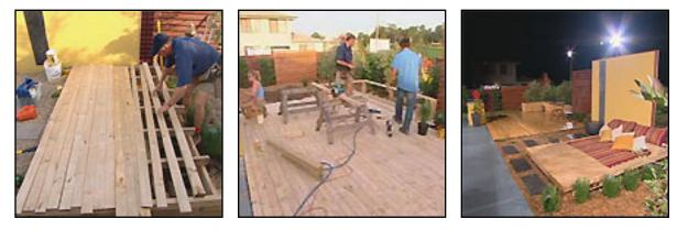
**Timber bench seats:** Scott built two long bench seats on top of the deck to provide seating and a sense of enclosure. Posts from the deck frame were extended through the decking to support a frame of bearers and joists. Decking boards were laid over this framework and nailed off with the decking gun.
