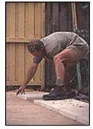
**Paving:** large reconstituted sandstone Classicstone pavers (500x500x40mm) were laid over compacted roadbase and paving sand. A fine grouting sand (Sydney sand) was swept through the gaps to bond the pavers together. Many of the pavers were cut using a bricksaw to house a tile (100x100mm) laid on mortar. The garden shed was placed on an area paved with concrete Besser block capping pieces (390x190x40mm). The paving was held in place with a mortar haunch around its edge.
