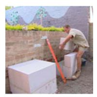
**Block seats:** Aerated concrete Hebel blocks (600x200x300mm) have been stacked to create formal seating between planted areas. A sand and cement footing supports the base course of blocks, while Hebel adhesive bonds the second course to the first. A coat of white exterior acrylic paint completes the formal seating. **Blitz Tipz:** Hebel blocks need to be sealed with a surface treatment to prevent them from absorbing moisture and deteriorating when they are used outdoors.
