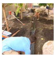
Water feature: two prefabricated pond shells (100mm wide, 6100mm long) were riveted together and painted with a waterproof, bituminous membrane. The shells were laid level in a sand-filled trench and surrounded by pavers (300x300mm) in a mortar bed. A sump with a galvanised metal grate houses the low voltage pump, which circulates water throughout the feature. Blitz Tipz: Only a licensed electrician can legally install a new powerpoint. Installation costs from \$200, depending on the location.
