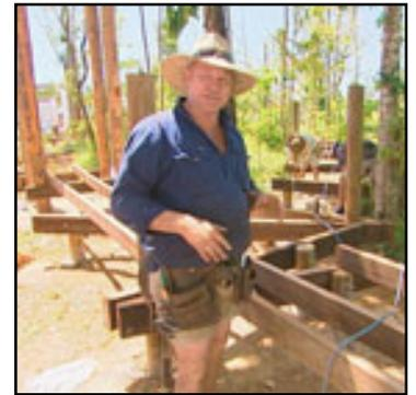
**Boardwalk:** All posts used in the boardwalk and stage area were either ACQ timber or hardwood. All bearers and joists were hardwood bolted to the posts and all decking was 30mmx140mm hardwood planks. This allowed us to span wider joist spacings.
