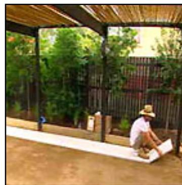
**Paving:** There are two sections of paving in the garden, a solid section laid on compacted crusher dust and a softer paving with mondo grass planted in between the pavers.
