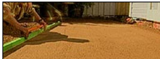
**Step 5** To begin the central feature lay the terracotta-coloured border and centre stones. A border paver cut into 100mm squares was used for the centre stones.
