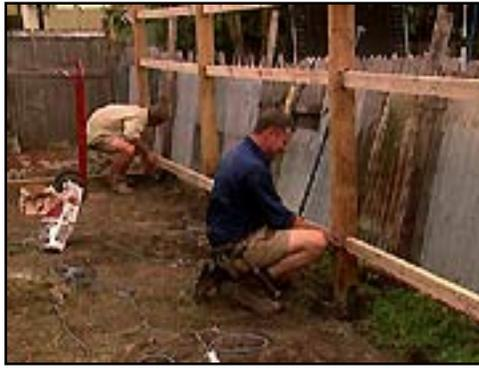
**Step 1** Before construction, paint the posts, cross rails, cover strips, capping and Hardiflex sheets.
