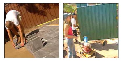
**Paved area with barbecue:** Jamie prepared the area for the sandstone flagging by using a 100mm depth of compacted roadbase and then laying each flagging stone on a 50mm wet bed of 4:1 sand cement. A rubber mallet was used to gently tap the flagstone level and into line. **Blitz Tipz:** To achieve a sandstone look in your mortar, use 4 parts of yellow brickies sand to 1 part off white cement.
