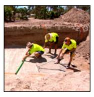
A cracker dust bed was screeded on the bottom of the excavation. The pool was craned into position and cracker dust was then poured in around the pool. At this point it is important to add water to the pool as we backfilled around the pool so as to retain the integrity of the pool shape. Once the pool was backfilled, and filled, a reinforced concrete capping was poured around the top of the pool edge and then the coping of pavers was glued to the concrete.
