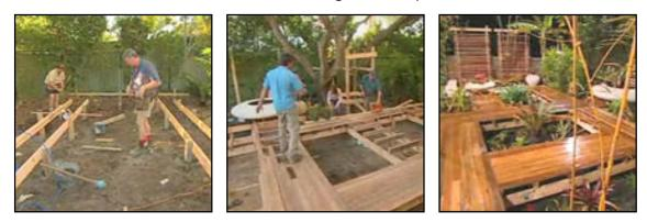
**Screens:** Jamie built decorative screens in the garden. He marked out screen locations and located post positions. H4 treated pine posts were concreted in ground using a spirit level to ensure each post was exactly vertical. Jamie then attached two lengths of rope to the top of each post and wove the rope around decking boards creatings a venetian blind effect. The end of each rope was then secured to the ground.
