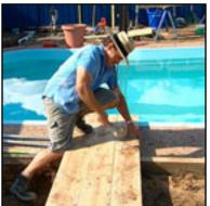
**Sleeper boardwalk:** Jamie and Scott built matching sleeper boardwalks on opposite sides of the swimming pool. Sleepers (2400x200x75mm) laid as bearers at right angles to the direction of the sleeper boardwalk provide a stable and level framework for the sleepers nailed above them. Galvanised decking spikes (150mmx9mm) were used to connect the boardwalk sleepers to the bearers. Once the sleepers were laid the ends were cut flush and straight.
