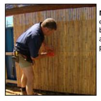
**Natureed and bamboo screens:** Jamie made some stylish screens to enhance the jungle theme by cladding the existing fence with Natureed and bamboo. Treated pine (70x35mm) screw-fixed to the metal fence provides a framework to attach the cladding. A finishing gun or electric stapler provides a clean neat finish and will hold the screens in place.
