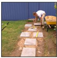
**Hopscotch:** Using a 4:1 mortar mix, Nigel laid concrete pavers in a hopscotch pattern. Jody painted numbers on each paver. The paver at the top section of the hopscotch game was cut with a wet demolition saw. *Blitz Tipz:* Use a paving paint appropriate for outdoor use on your hopscotch court.
