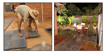
pattern over a compacted subgrade of roadbase and coarse washed river sand. Grouting sand swept through the pavers helps to bind them in place, while a 4:1 mortar haunch prevents bedding sand from washing away.
