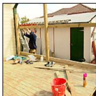
Decking boards were nailed over the angled bearers to complete the ramp. Posts at one end of the deck were continued beyond deck height to support rails (70x35mm). These had pine fence pickets attached to create a decorative screen.
